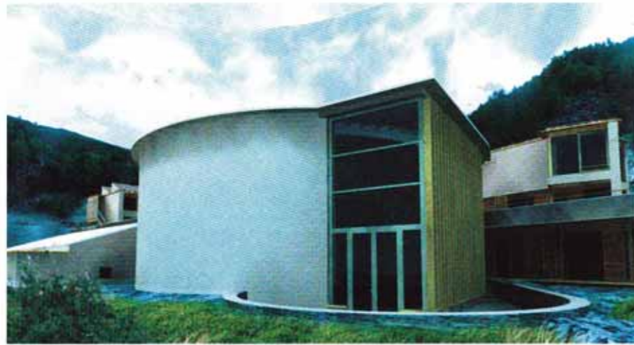
Right: the 200-seat lecture theatre will feature a self-supporting, double-skinned roof
